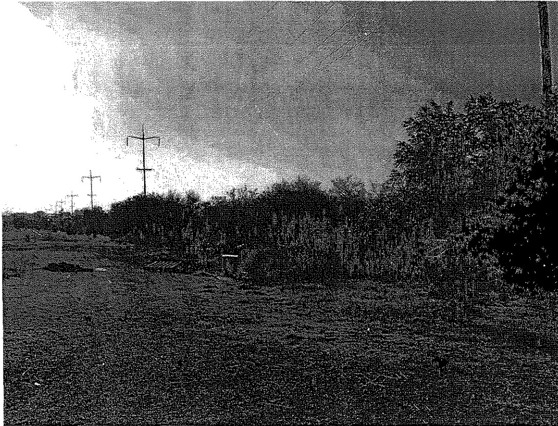
Photo 4 - Unusable parcel size at the point of the railroad spur triangle.
